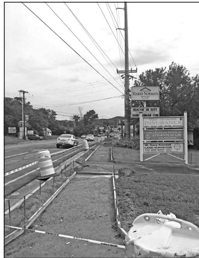
Construction of the brand-new sidewalk on Hiwassee Main Street.
